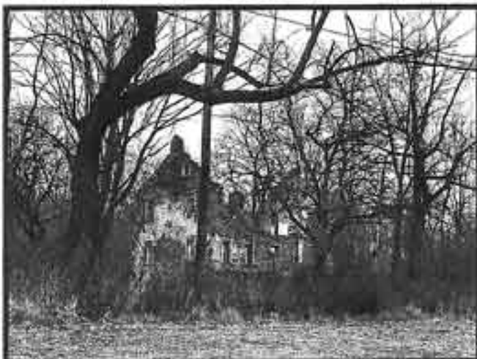
This late 1700's house stood intact on the Ulmer property until the mid 1980's, when a careless tenant let the potbelly stove overheat, burning the structure beyond repair.
