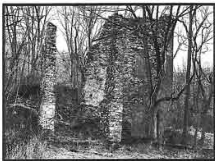
Ruins of yet another 1700's structure located elsewhere on the property. Once again, a 20th century fire was the culprit that brought the historic building to the ground.
